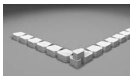
Start outside corner with a half unit.
