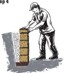
**Step 4** - On the last course of stacking units, remove locating lugs on top of the Versawall™ blocks, place a line of adhesive front and back and place the capping unit. Apply pressure to secure and use a stringline and level for the best result. (See Pic 3A and 3B)
