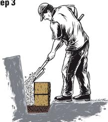
**Step 3** - Fill Versawall™ cores and 300mm behind each course with granular rock for drainage and carefully compact. Check each course is level before proceeding and stacking each additional row offsetting from the block below to maintain half bond.
