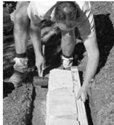
**Handy Tips:** Use a rubber mallet to tamp blocks into place – a metal hammer may crack them.
