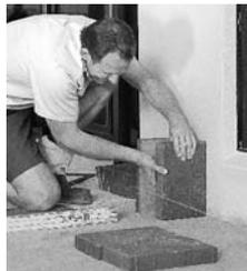
**Handy Tips:** Keep close to the ground (not arched over) when laying pavers to protect your back.
