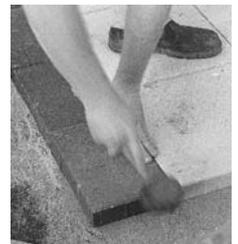
**Handy Tips:** An old piece of carpet under the compacting plate will avoid chipping any pavers.
