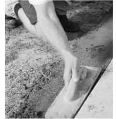
**Handy Tips:** For a neat job, trowel the excess concrete up against the paver at a 45 degree angle.
